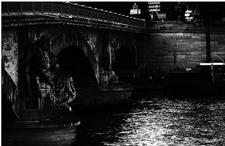
Alma Bridge, Paris, France, by Guyomar Pillai
