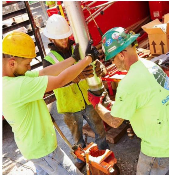
Geothermal well drilling for the Center for Computing & Data Sciences. September 2019. Photo: Dave Green Photography.
