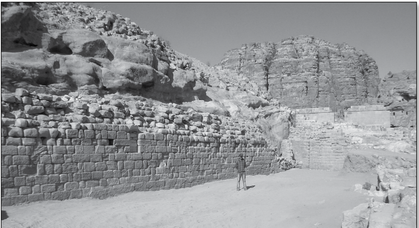
The South Wall forms a backdrop to the PGPC pool complex.
