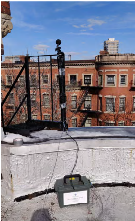
Photo 3: SLM at Location 3
