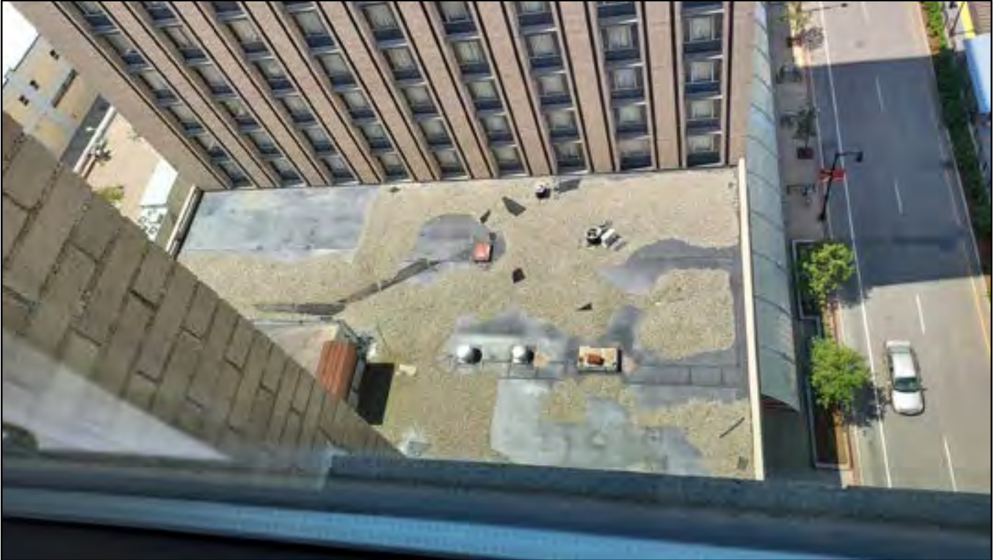
Photograph 6: Elevated view from Tower B looking west at Podium Roof C.
