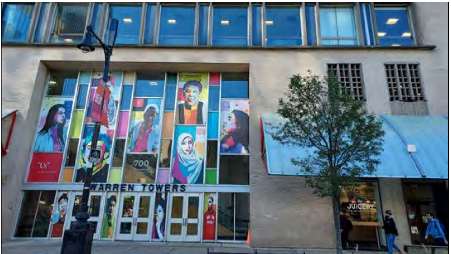
Photograph 2: View from Commonwealth Avenue looking south at Project Site front entrance.
