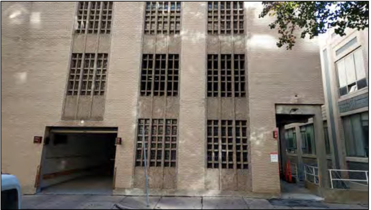
Photograph 3: View from Cummington Mall looking east at Project Site garage entrance.
