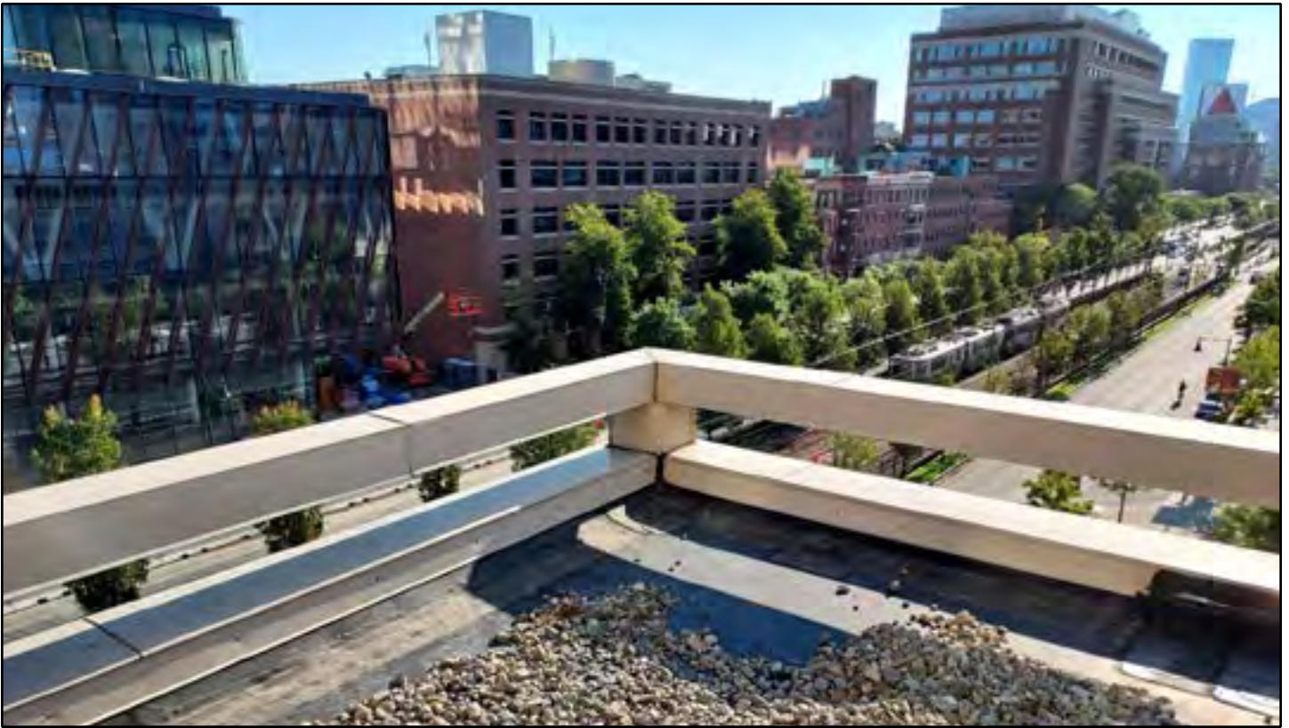
Photograph 5: View from Podium Roof A looking east at Commonwealth Avenue.
