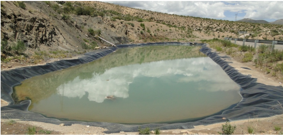
PICTURE 4: AGUA DULCE WATER SUPPLY SYSTEM, POTOSÍ - BOLIVIA
