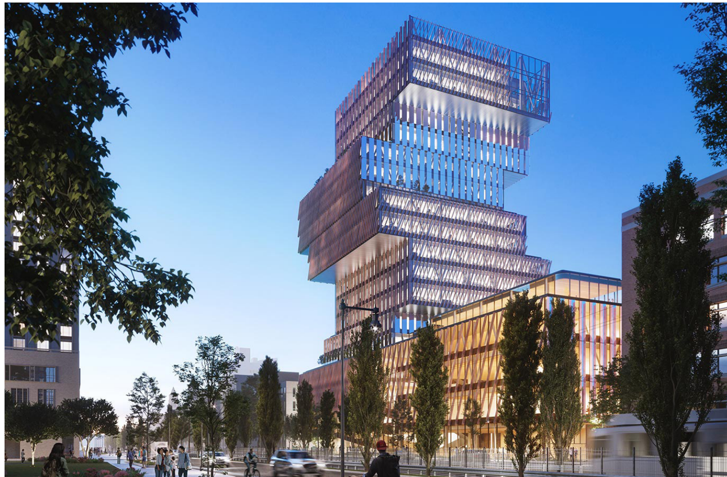
Mock-up of the new Center for Computing & Data Sciences, which will house the Hariri Institute for Computing
