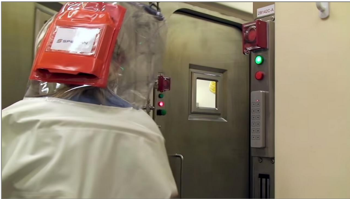
A scientist walks through the first air pressure resistant (APR) door at a biosafety level 4 (BSL-4) laboratory Credit: NIAID
