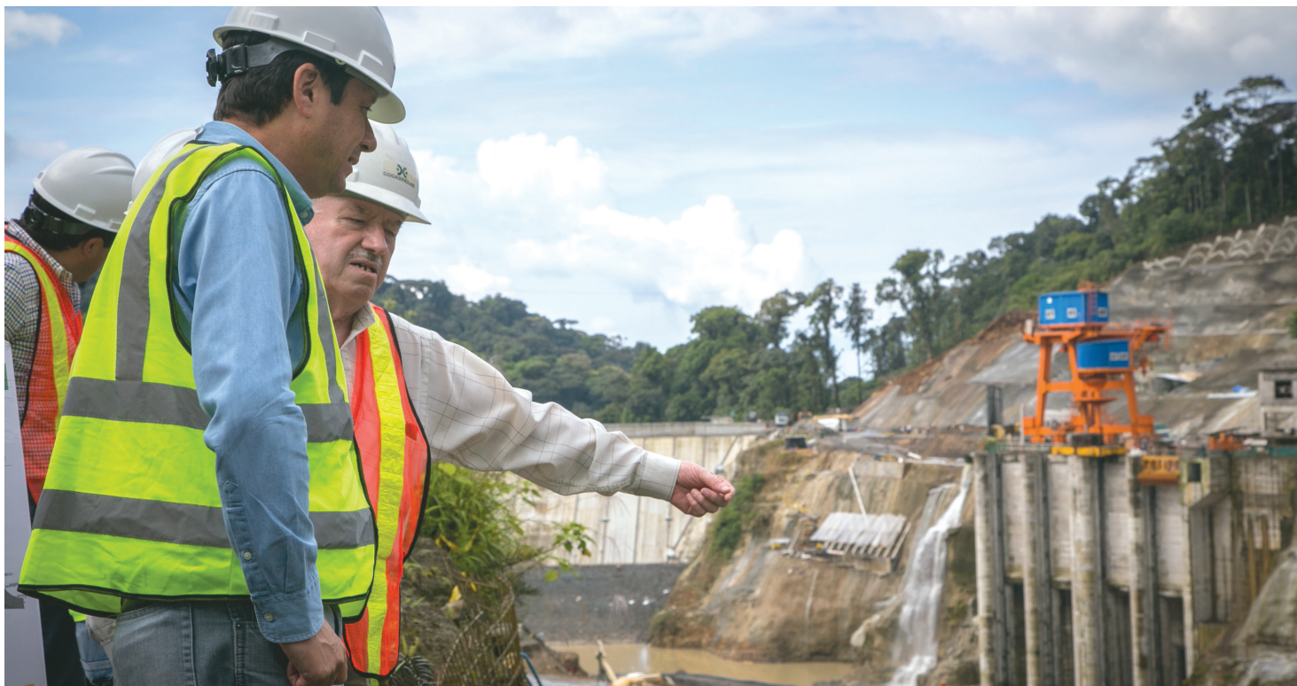
Ecuadorian Minister of Electricity and Renewable Energy Esteban Albornoz, foreground, visits the Coca Codo Sinclair hydroelectric project. (Photo courtesy of Ecuadorian Energy Ministry)
