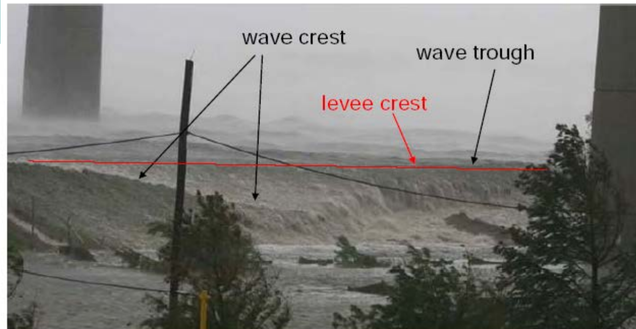
Figure 15-39. Photograph showing overtopping of levee under the Paris Road Bridge. Time of the photo is not known with certainty. View is from the north side of the levee, looking towards the southwest. Waves are traveling from the east (left side of photo) towards the IHNC
